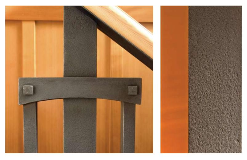
ABOVE: A detail of the railing rivets echoes the precise, geometric design of the steel balustrade. We etched the surface of the metal to expose the crystalline structure of the steel.
